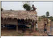
Almost there - finishing off the roof.
